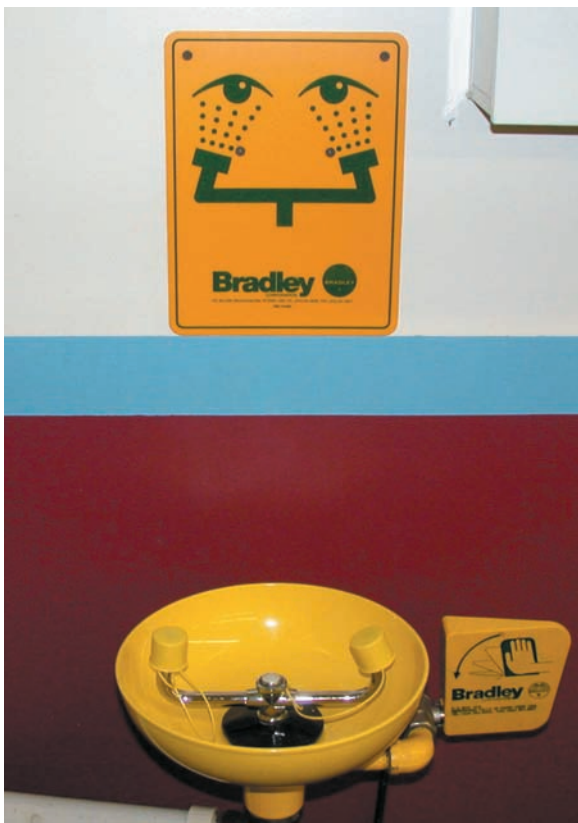
FIGURE 1-16 A typical eye wash station. Often a thorough flushing of the eyes with water is the best treatment in the event of eye contamination.
