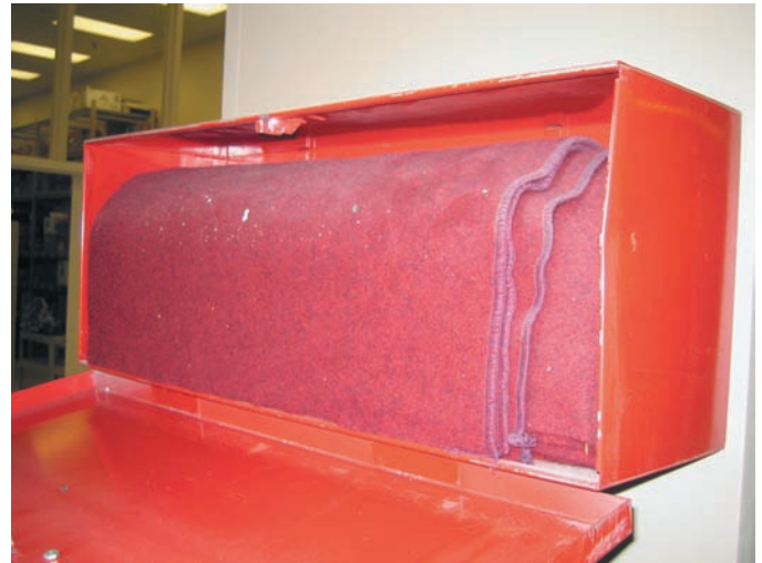
FIGURE 1-14 A treated wool blanket is kept in this easy-to-open wall-mounted holder and should be placed in a centralized location in the shop.
